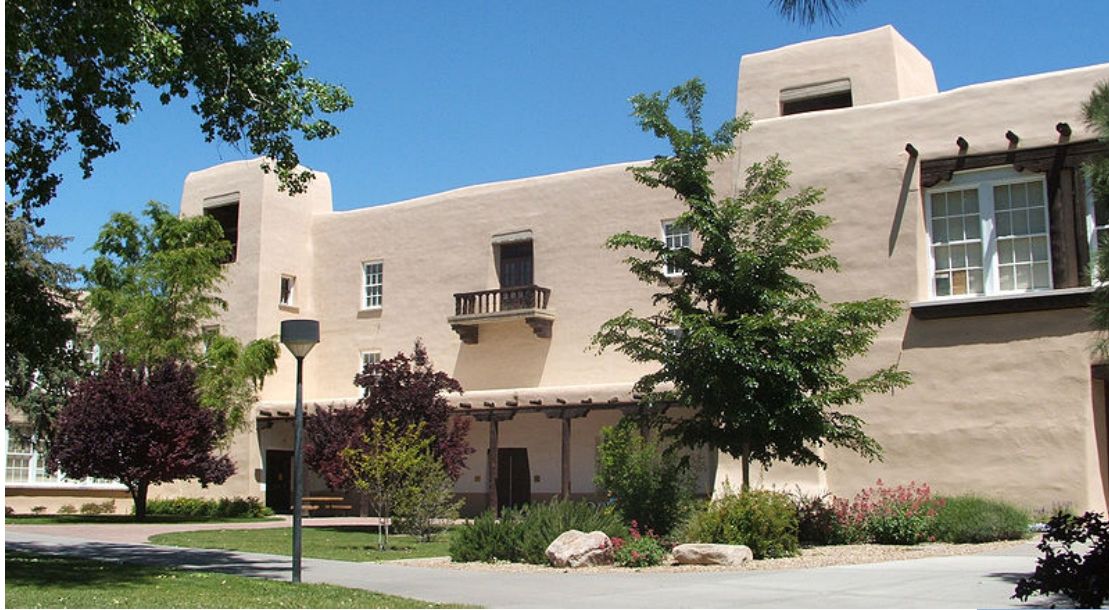
John Gaw Meem, Administrative Building (now Scholes Hall), 1934-1936. University of New Mexico, Albuquerque, NM.
