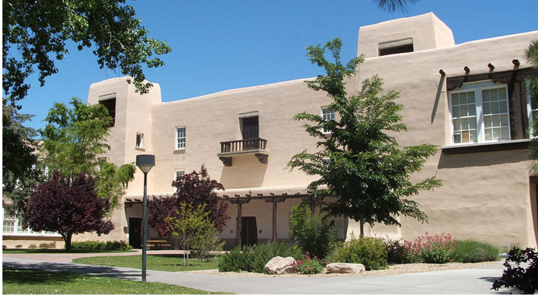
John Gaw Meem, Administrative Building (now Scholes Hall), 1934-1936. University of New Mexico, Albuquerque, NM.
